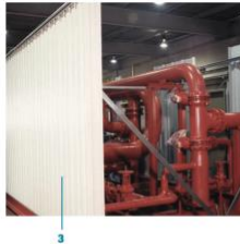
This system includes three electric motor driven fire pumps, 16' x 53' and weighs 57,000 lbs.
